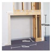
Timber framework partially clad with 18mm Villa Board
